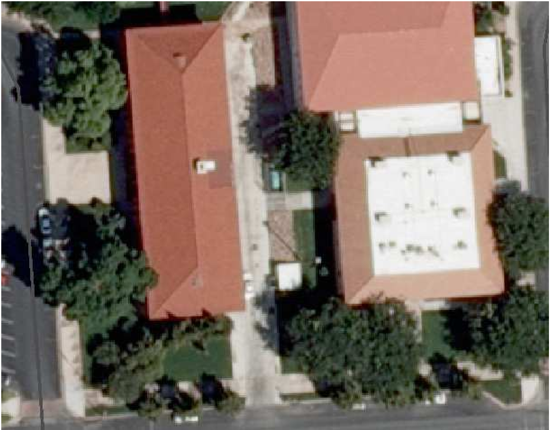
CITY HALL & PARKS & REC BUILDINGS
